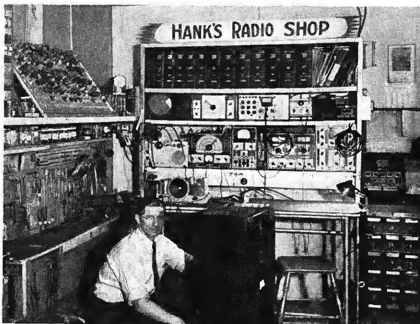
H. W. Attebery, manager of Hank's Radio Service, 723A Seventh St., Greeley, Colo., cut servicing time by one-third using this arrangement. A movable work bench, and parts within easy reach facilitate this technician's work.
